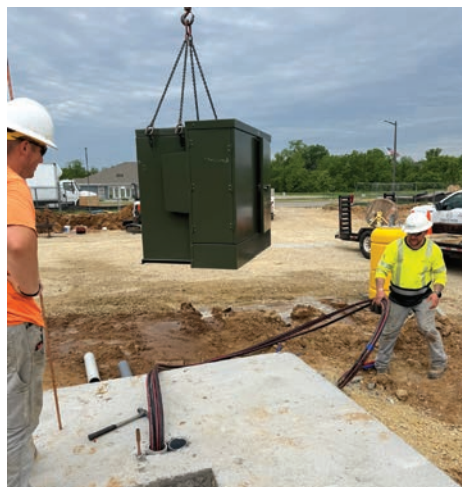
Left: Underground conduit and primary electrical cable are installed before the pad-mounted transformer is set in place at the new Kwik Trip in Ellsworth. Right: Foreman Aaron Langer (left) and Apprentice Lineman Tucker Ingenthron guide a pad-mounted transformer into position.
