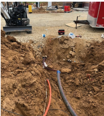
Left: Underground conduit and primary electrical cable are installed before the pad-mounted transformer is set in place at the new Kwik Trip in Ellsworth. Right: Foreman Aaron Langer (left) and Apprentice Lineman Tucker Ingenthron guide a pad-mounted transformer into position.
