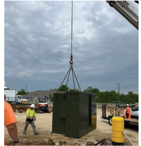
Foreman Aaron Langer and Apprentice Lineman Tucker Ingenthron work with the crane operator to carefully position a pad-mounted transformer during construction.
